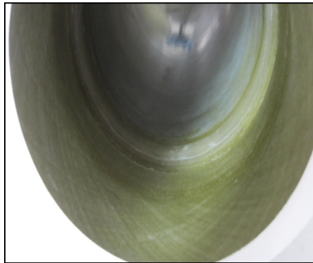
Figure 2.9 Inspecting the vessel
